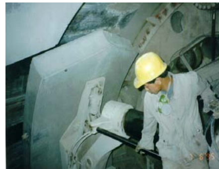
Figure 4: Honeycomb segmental lining for water supply tunnel on WYRDP in PR China in 1998 [2].
