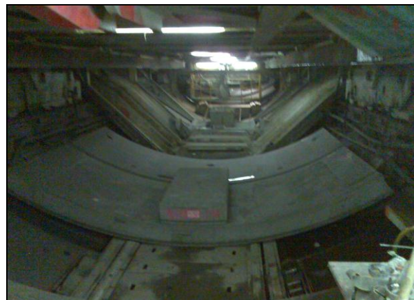
SEGMENTAL LINING READY FOR INSTALLATION
