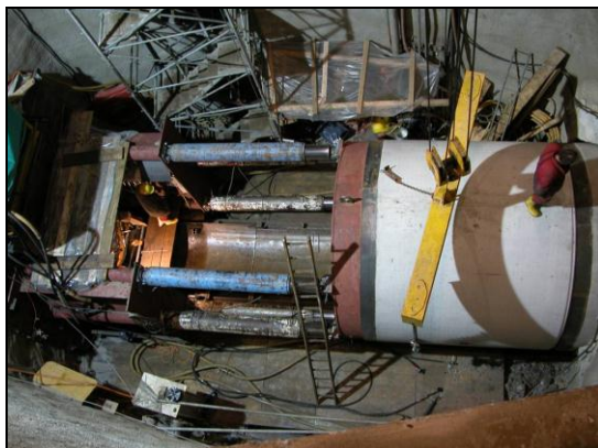
PIPE JACKING FROM START SHAFT
