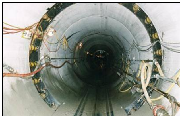
STRETCHING UNIT FOR INTERMEDIATE PIPE JACKING
